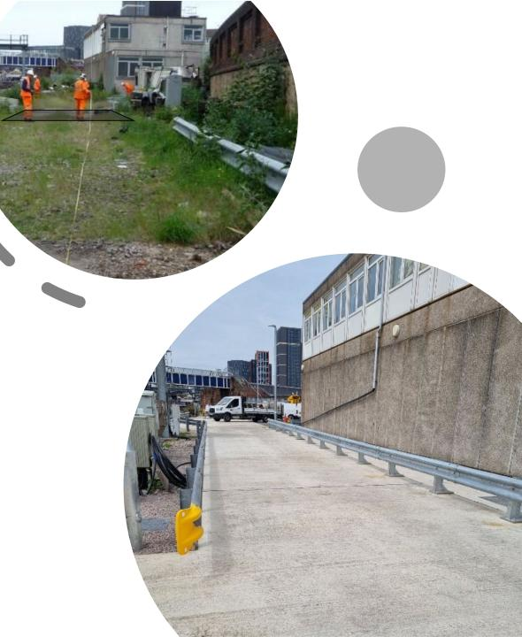
Over a 12-week programme Seva Rail successfully carried out clearance works, de-vegetating the area to allow the works to start. First to secure the site we installed 1.8m high palisade fencing with new double gates and set to work on the groundwork including new drainage, sub-base, kerbing and vehicle barriers as per the supplied design.
